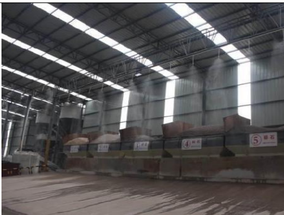
拌合场站内喷淋
