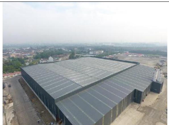
拌合站全封闭
